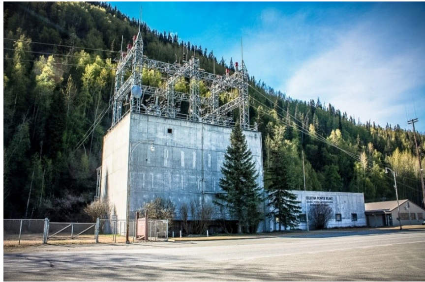
Figure 2-3. Eklutna Power Plant.
