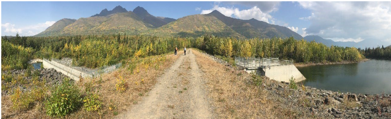
Figure 2-1. Dam crest and ungated overflow spillway, looking north.
