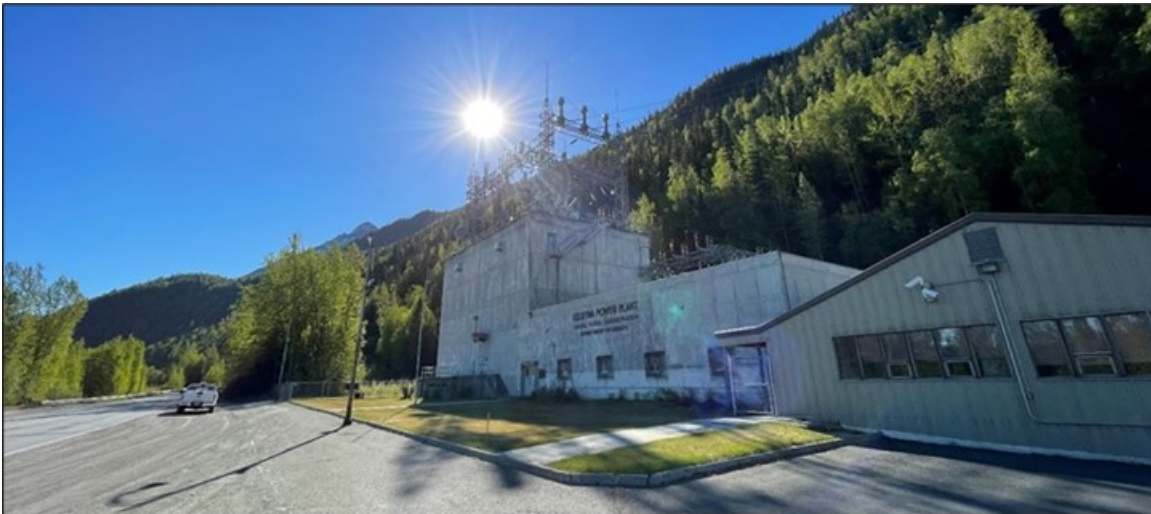
Figure 3.2-1. Eklutna Powerplant as Viewed from Old Glenn Highway.
