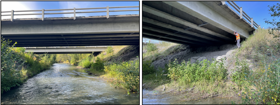
Figure 4.3-1. New Glenn Highway Bridges D/S View (Left); Right Abutment (Right).
