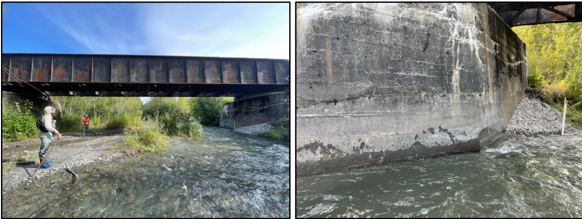
Figure 4.4-1. Eklutna River Railroad Bridge U/S View (Left); Left Abutment Wall (Right).
