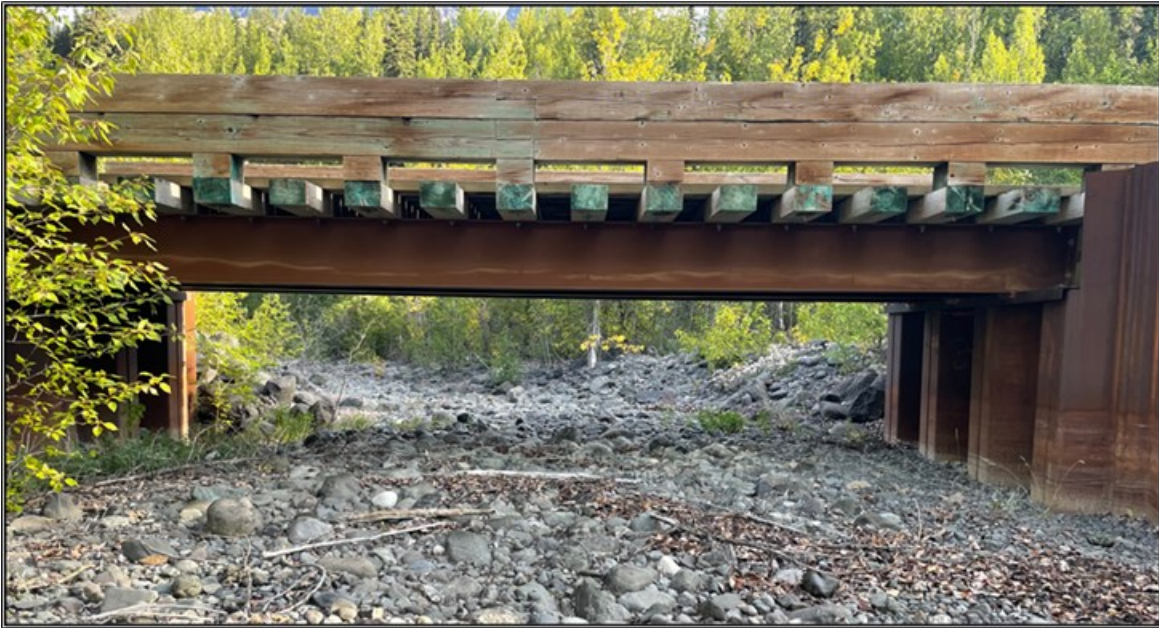
Figure 4.1-7. AWWU Bridge No. 1; Looking Upstream.
