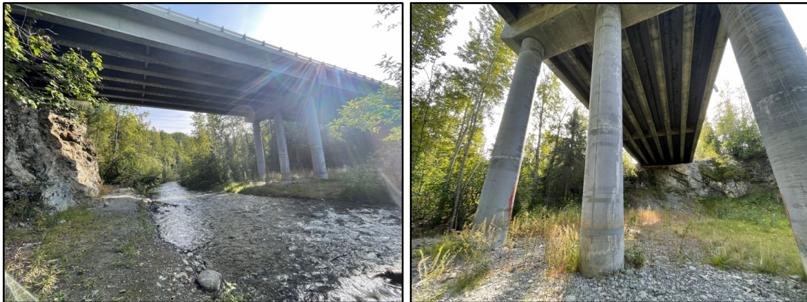
Figure 4.2-1. Old Glenn Highway Bridge U/S View (Left); Bridge Pier (Right).
