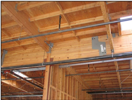
Solid sawn or glulam construction
