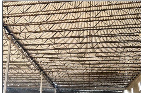
Open web steel truss
