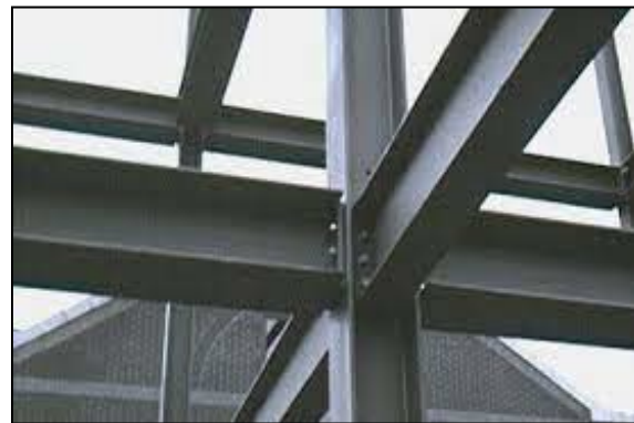
Structural steel framing
