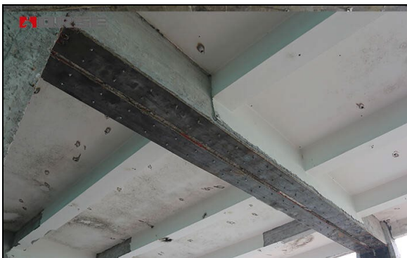
Solid concrete construction
