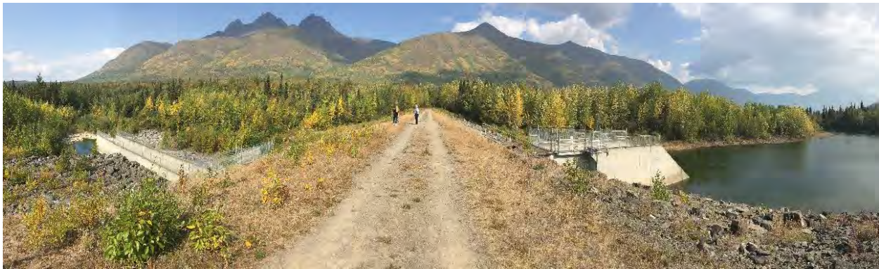
Figure 1-2. Dam crest and ungated overflow spillway, looking north.
