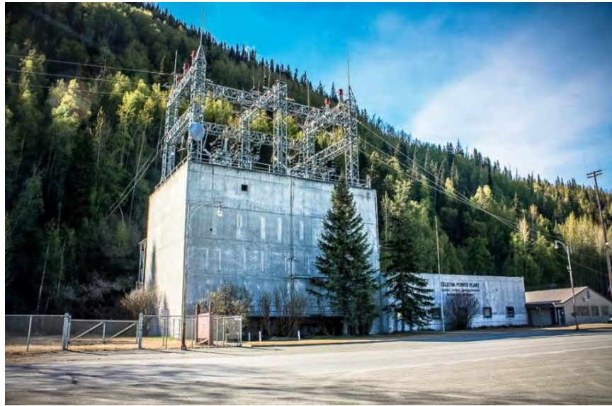
Figure 1-4. Eklutna Power Plant.
