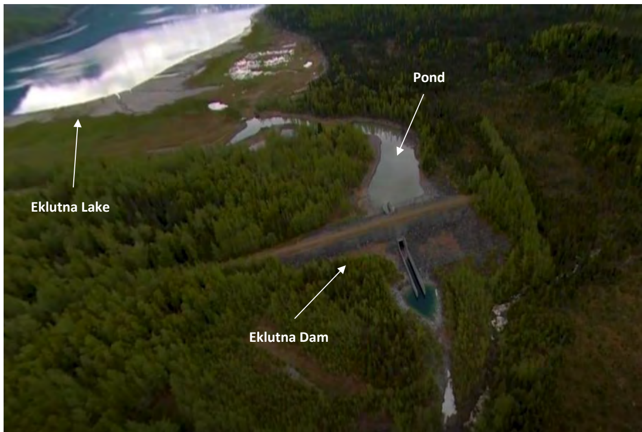
Figure 1-3. Pond between the natural glacial moraine and existing dam in May 2020.
