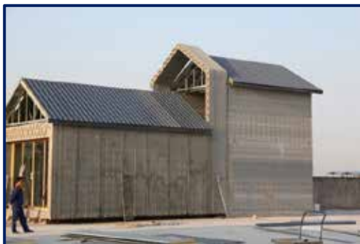
Ten 3DCP Square Houses Built in 24 hours; 2014
