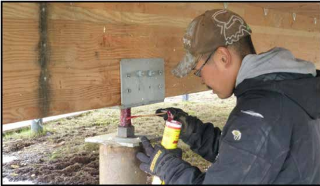
Figure 27. Saddle bracket jack
