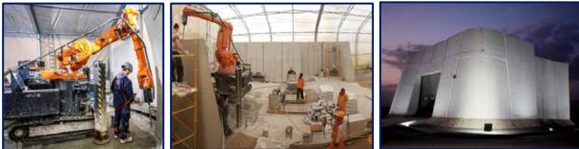
Figure 27: Images and Summary of CyBe 3D Construction Printer Characteristics
