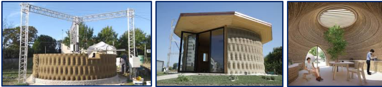
Figure 34: Images and Summary of WASP Printer Characteristics
