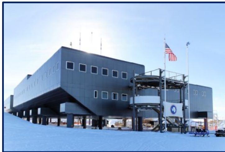
Figure 8: U.S. NSF Research Center in Antarctica On Pilings
