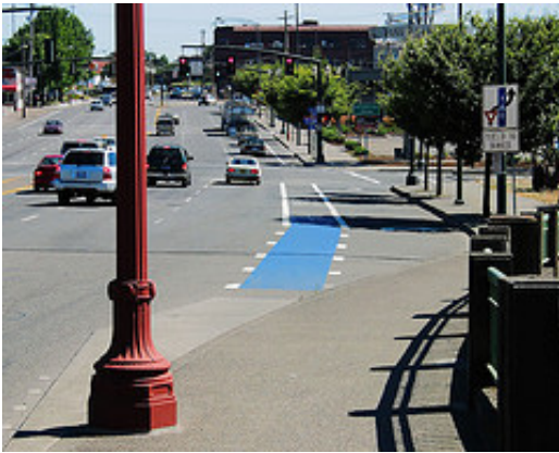
Bicycle lane treatment at a right-turn-only lane
