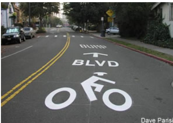
An example of a local street marked as a bicycle boulevard (Portland, Oregon).
