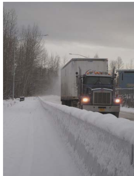
42-inch concrete separation – Ship Creek Trail at Viking Drive
