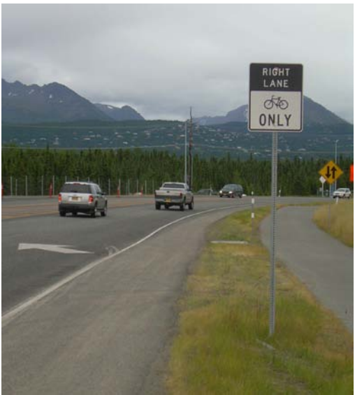
Bicycle lane – Elmore Road
