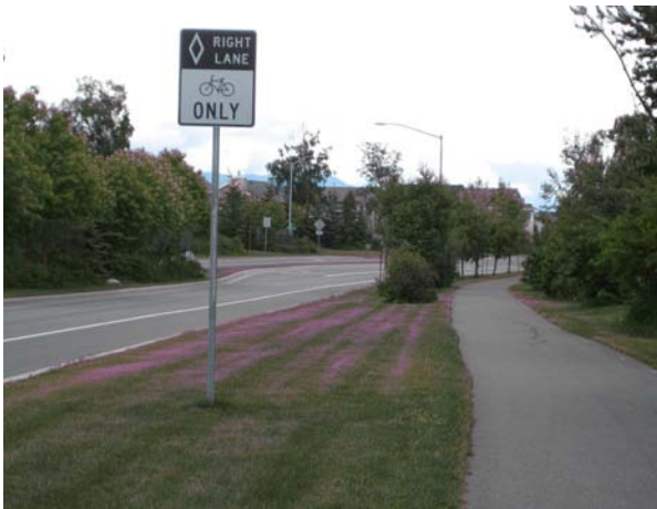
Bicycle lane and separated pathway – Southport Road
