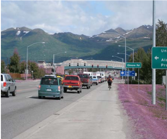
Back-of-curb pathway – Tudor Road
