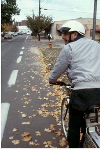
Bicycle lane with debris
